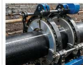
Fusion Welding HDPE Joints
