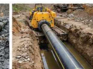
Trenchless Installation & Pipe Bursting
