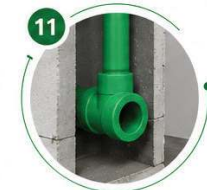
Concealed installations in wall cavities
